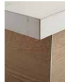
5.6mm Back Mitered and Epoxied
