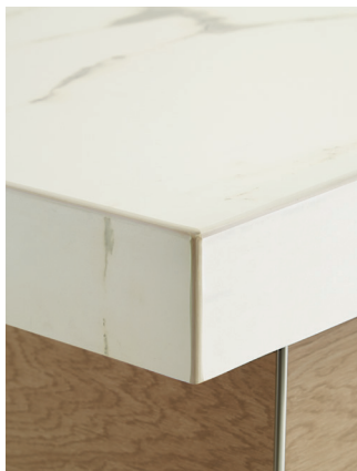
5.6mm Field Applied Bullnose
