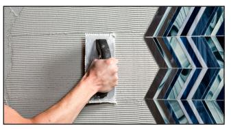
**Step 2** To establish the proper depth of the setting bed, use a 3/16" x 1/4" v-notch trowel to apply additional thinset and comb full notches in one direction.
