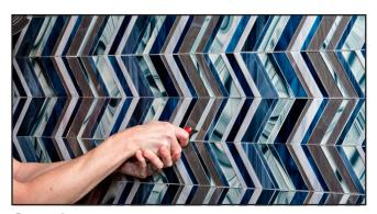
**Step 6** If necessary, remove excess thin-set from the grout joints with a razor knife prior to grouting.
