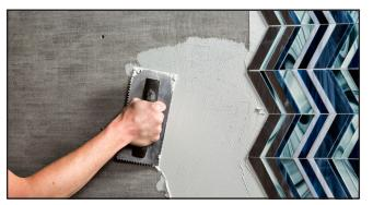
**Step 1** To initiate the bond coat, use the flat side of a trowel and firmly apply thin-set to the substrate.
