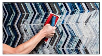
**Step 7** Apply grout per the grout manufacturer's instructions. When grouting with sanded grout, use care during application to minimize scratching.
