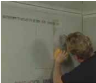
Mark and cut area for Niche
